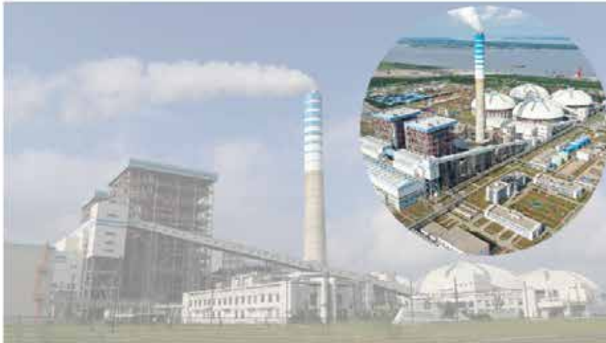
Eco-friendly Ultra-Supercritical Technology implemented Power Plant Payra 1320 MW Thermal Power Plant (1st Phase)
