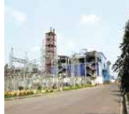
Raozan 25 MW Dual-Fuel Power Plant
