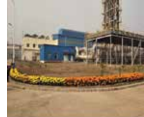
Gazipur 105 MW HFO Fired Power Plant
