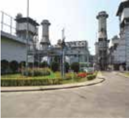
Mymensingh 210 MW Power Station
